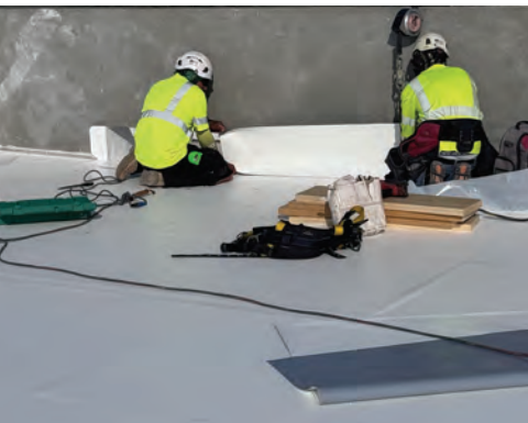
A roof champion observed these workers installing through-wall scuppers.
