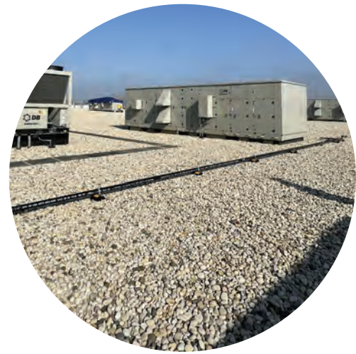
Existing ballasted roof assembly that a roof champion reviewed for roof deflection
