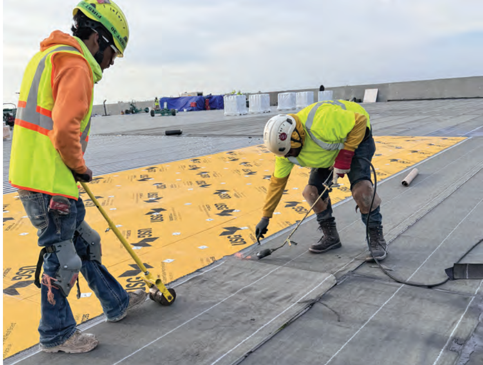
A roof champion can observe torch-down vapor retarder installation.
