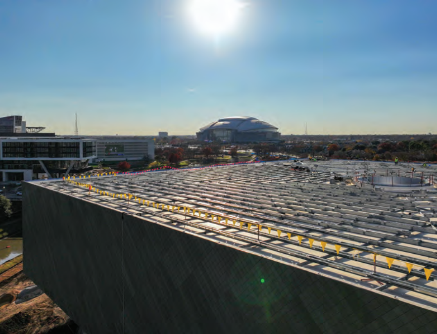
Hundreds of steel penetrations on the exhibit hall roof required meticulous attention to detail. Newly constructed National Medal of Honor Museum
