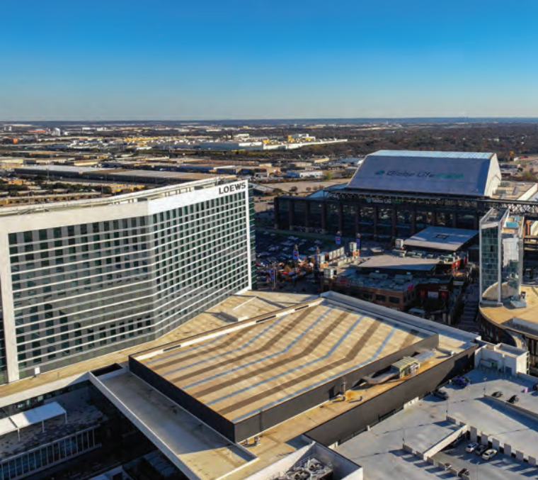
Completed pumphouse roof
