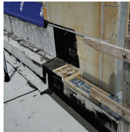
A roof champion reviewed the construction detailing at this parapet interface.
