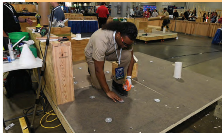
Dominic Rodriguez from Florida installs insulation.
