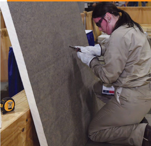
Karley Wickman from Iowa installs insulation.
