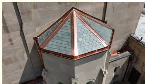
Top to bottom: Aerial view of new slate roof system; 18- by 10-inch slate tiles were used on all upper steep-slope areas; for the lower roof, 20- by 10-inch tiles were used.
