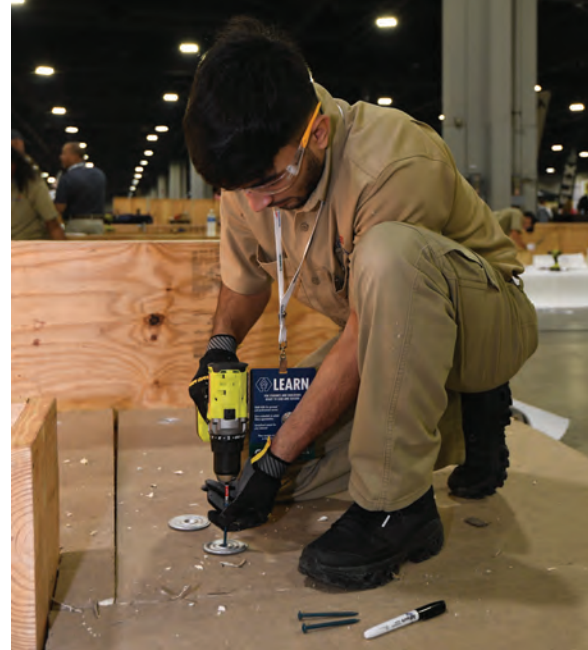
Alberths Figueroa from Texas installs insulation.
