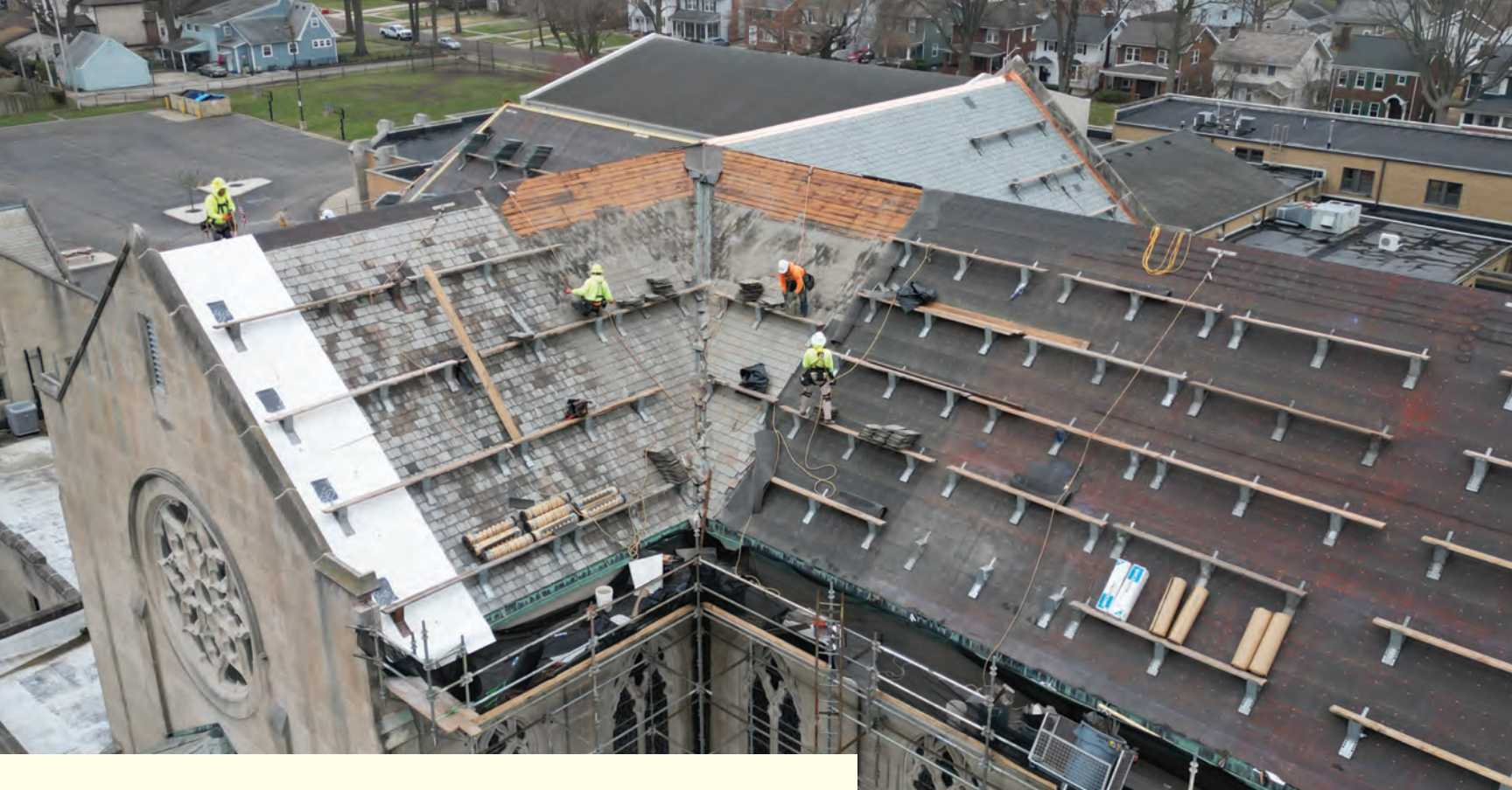
The church roof under construction
