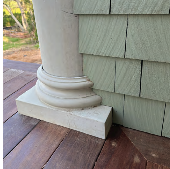
For the siding, the team installed shingles stained Orchard Green and included varying insertions of custom-cut shingles.
