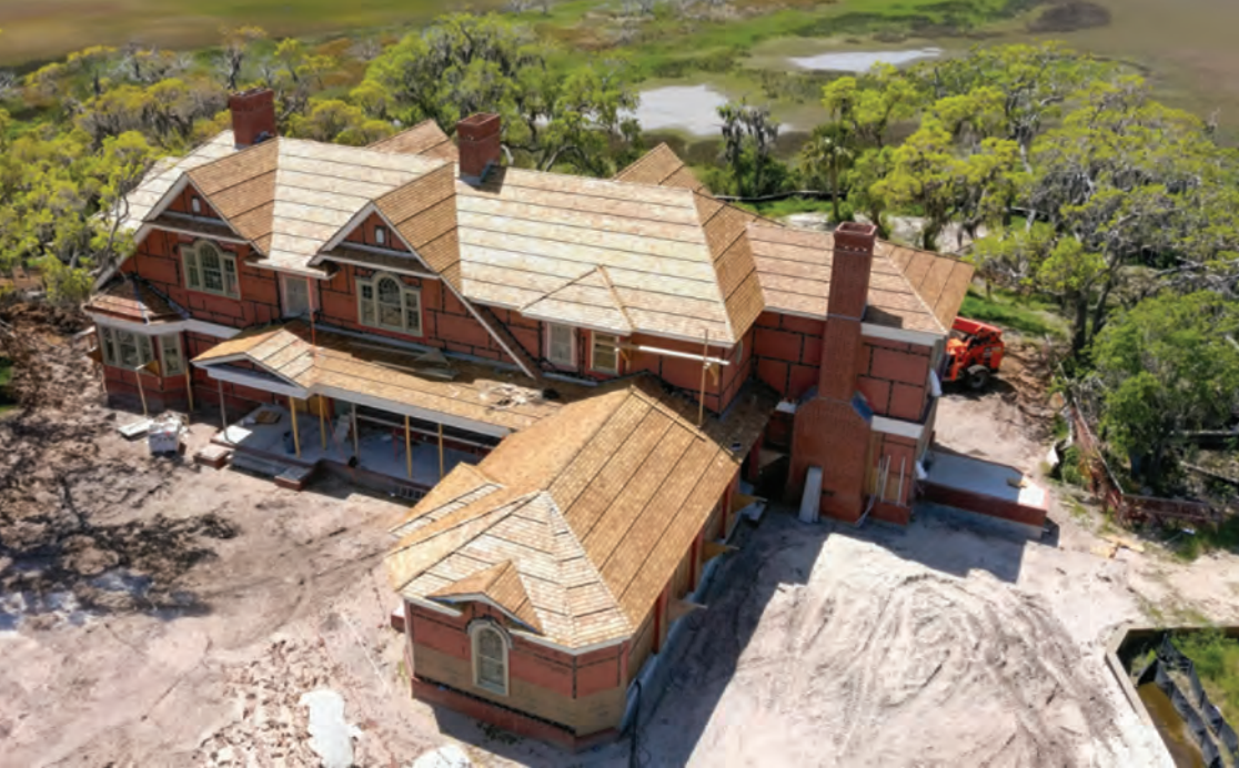
Aerial view of completed roof system
