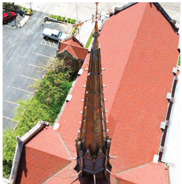
Aerial view of the completed steeple
