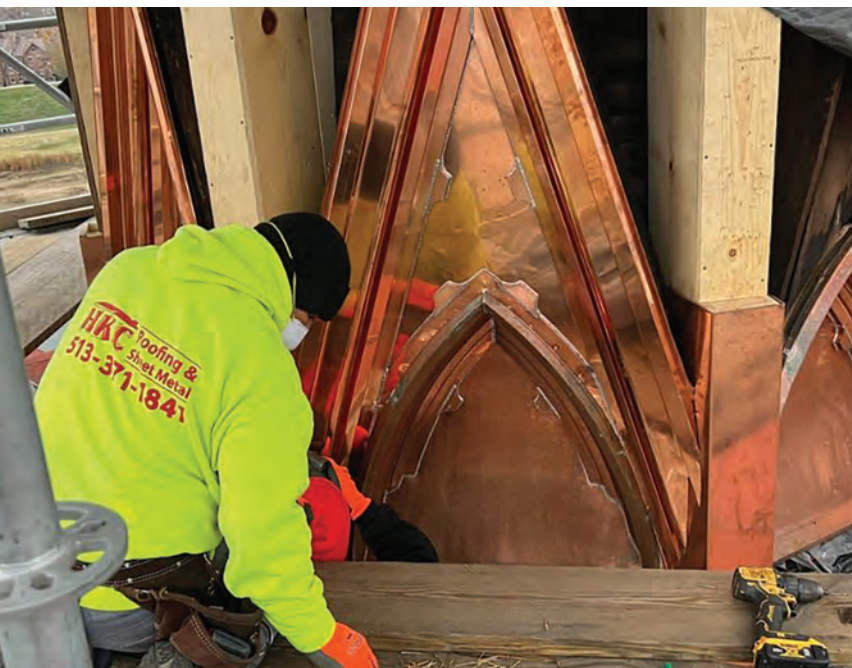
All copper components were fabricated by hand from 20-ounce copper.
