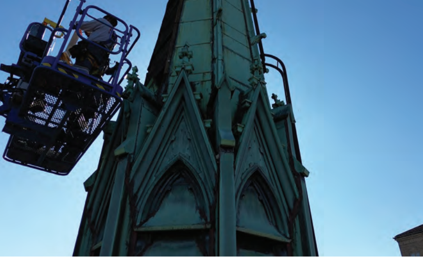
Crew members remove copper cladding and decorative elements.
