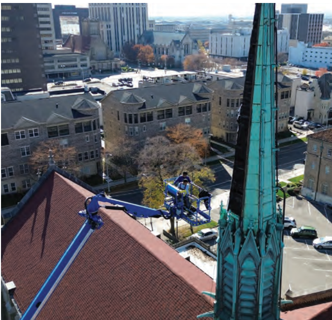
The project called for surgical removal and replication of copper elements.
