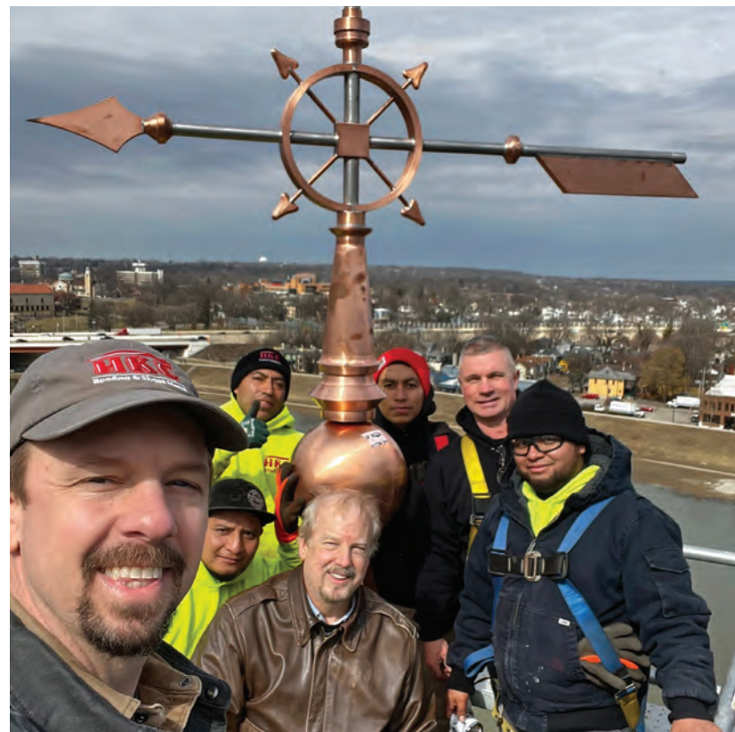
The HKC Roofing and Sheet Metal crew completed the steeple with a weathervane.
