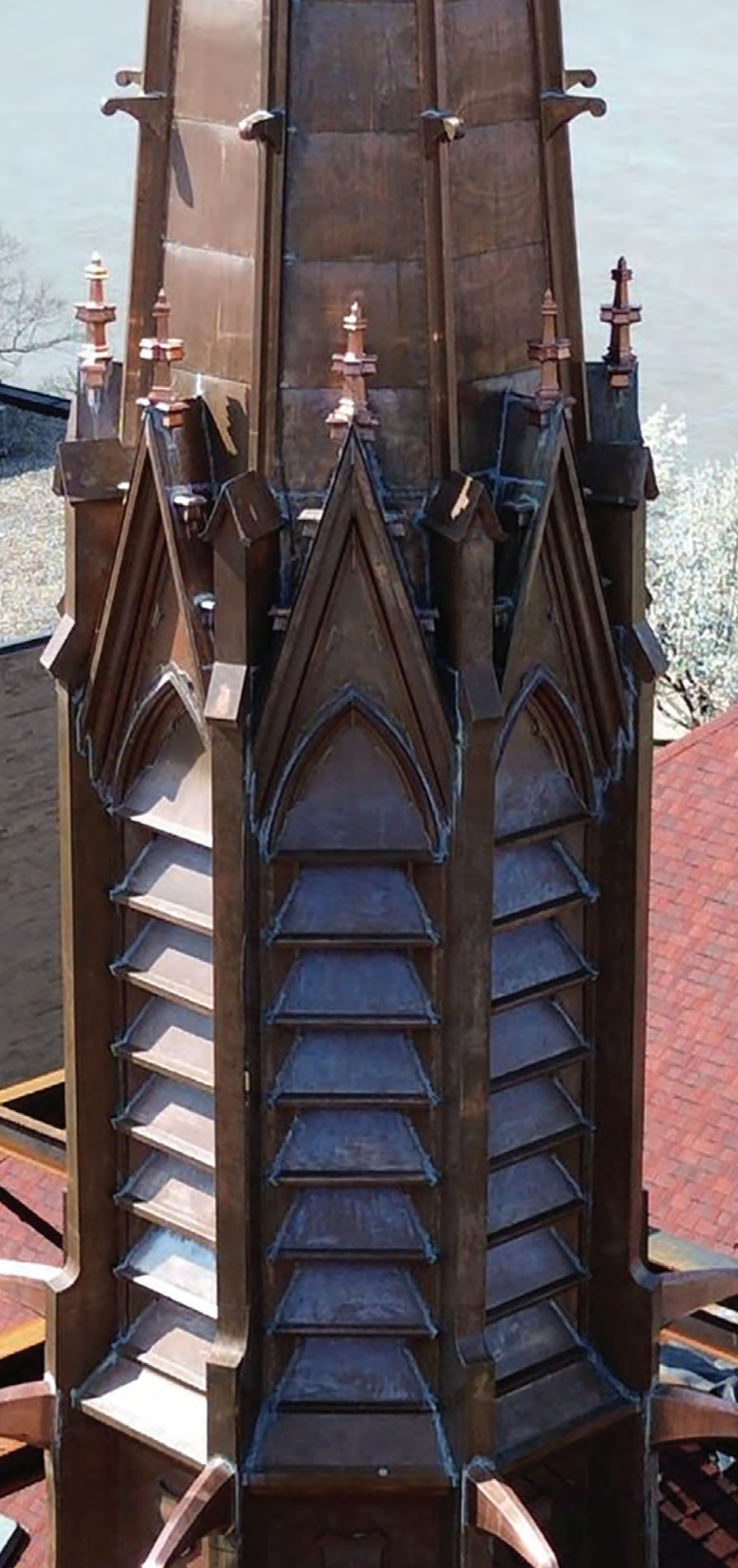
The steeple after restoration
