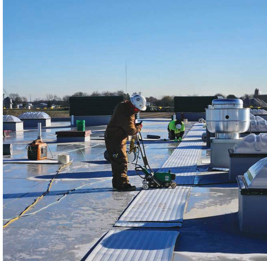
New roof system in progress
