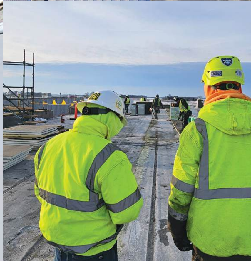
Crew members assess roof areas
