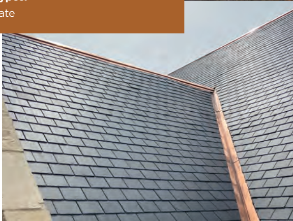
Left and above: Thousands of slates were installed on the courthouse roof.
