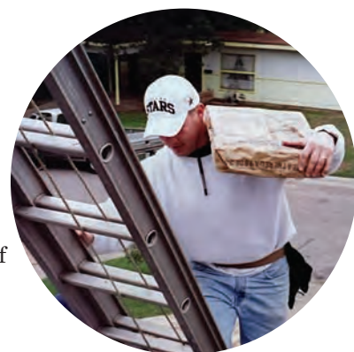
As part of his training, Sanders had to install a roof system.
