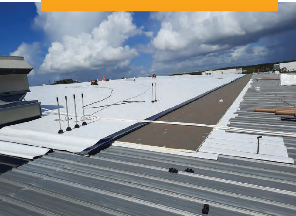
The roof system layers on the new building
