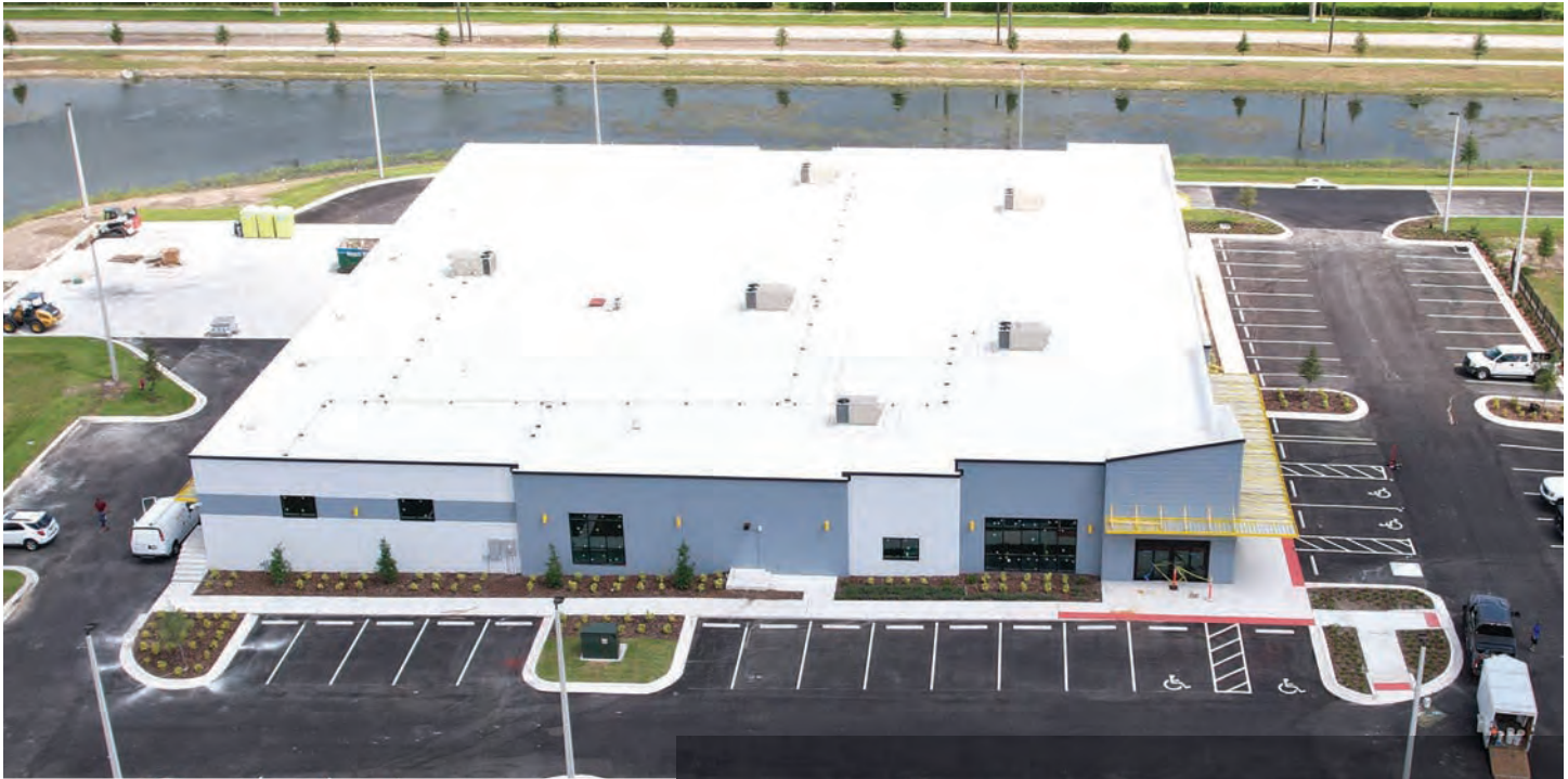
Aerial view of the new roof system on the existing facility
