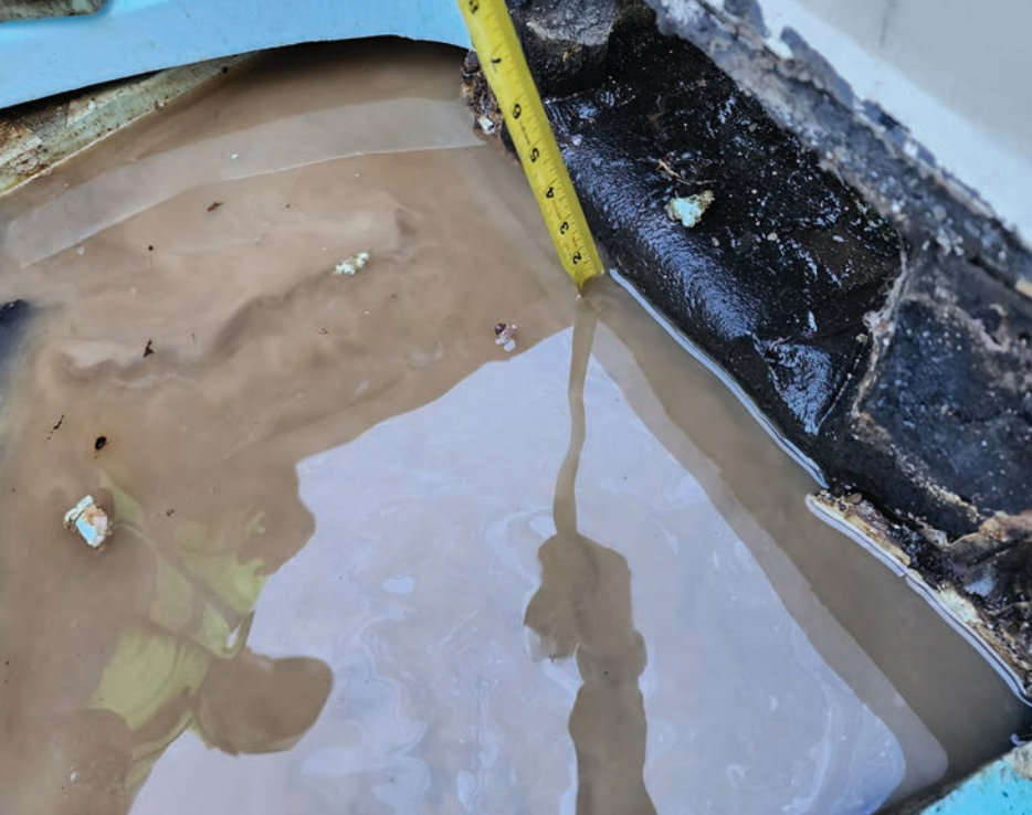
Flat decks are never truly flat; water collects at low points and lingers below the surface.
