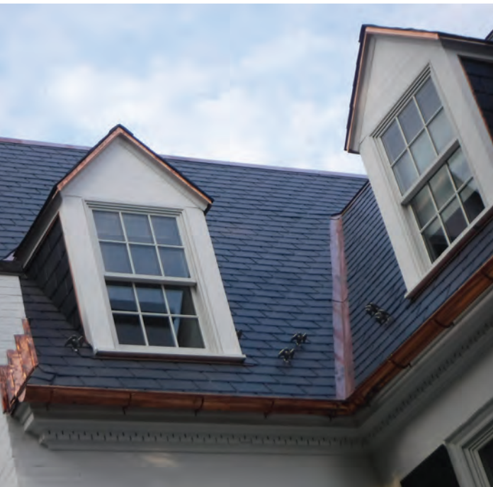
New roof with synthetic slate
