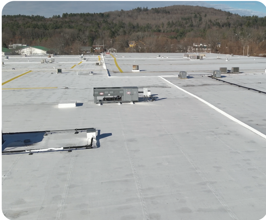
Drone view of newly completed roof
