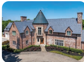
Great Roofing & Restoration's project
