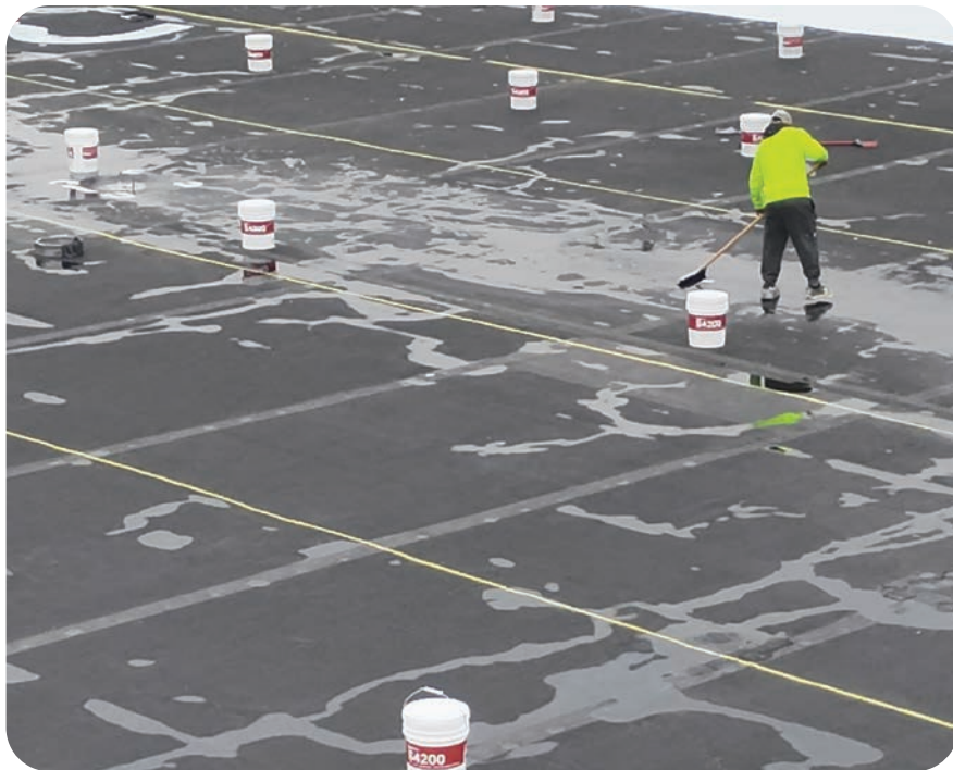
A Certified Roofing Systems crew member at work
