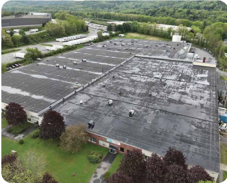
Old EPDM roof
