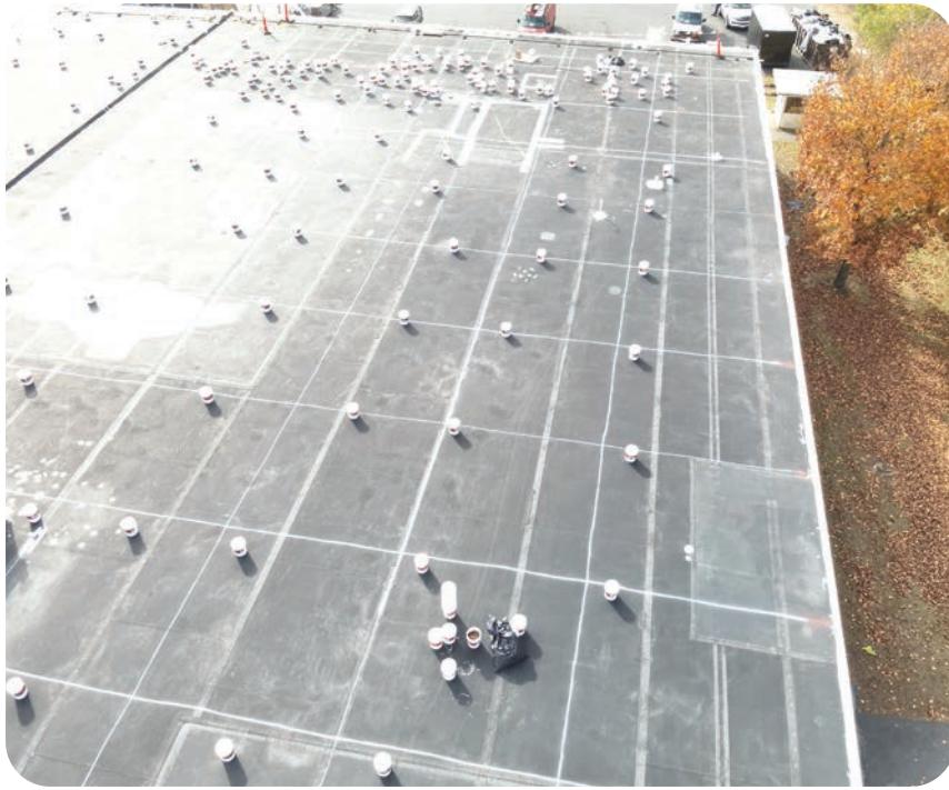
New roof in progress
