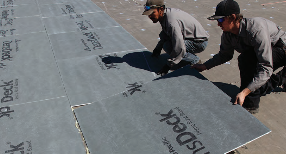
Using a cover board on a single-ply membrane roof can increase the median life expectancy by four years.
