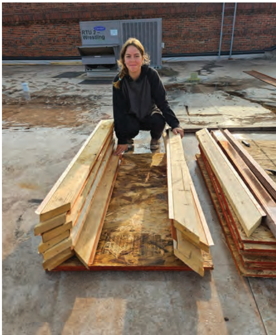
New wood battens for the copper panels
