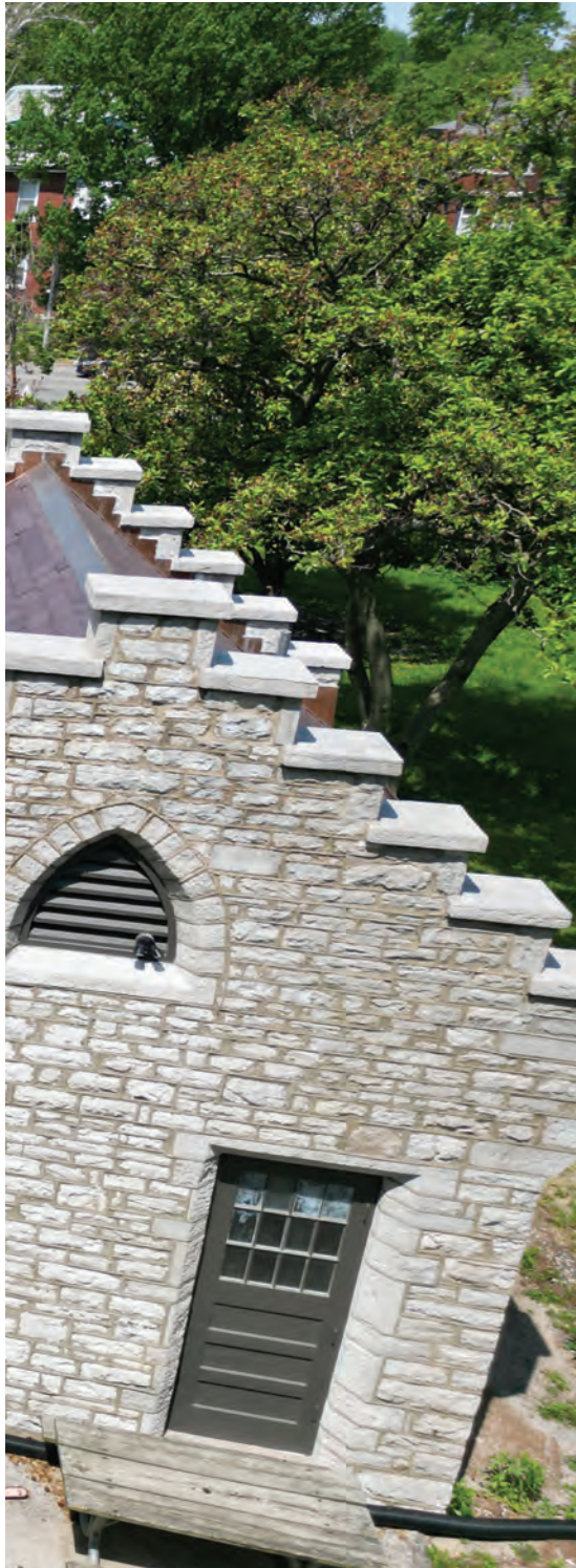
Tower Grove Park West Gatehouse's new roof system
