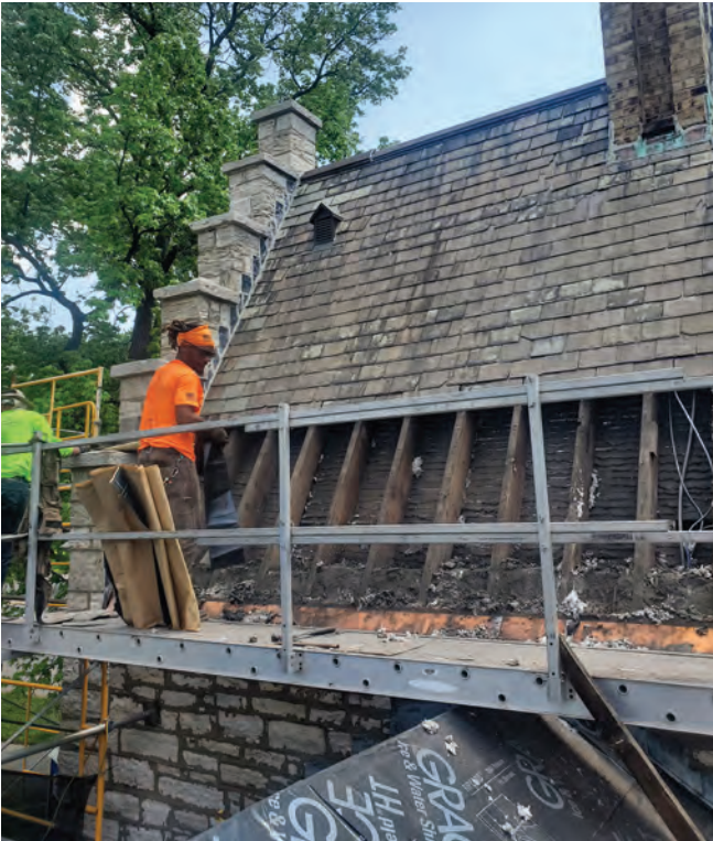
The slate roof area during construction
