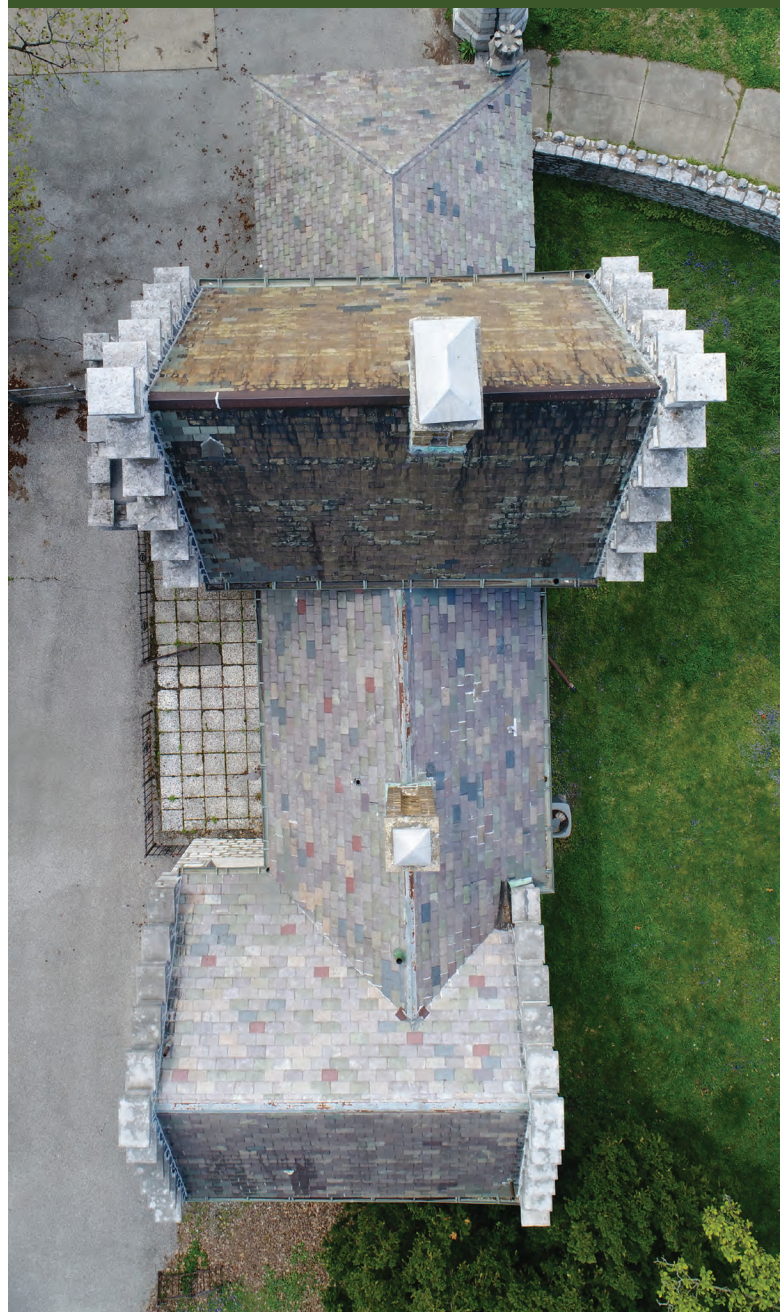
Aerial view of roof areas before renovations
