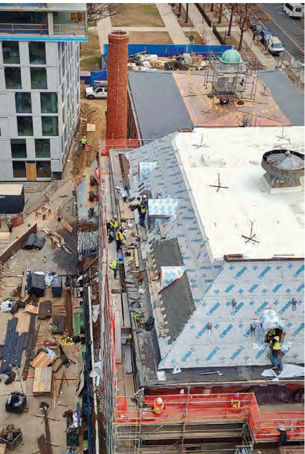
Aerial view of the new roof systems under construction
