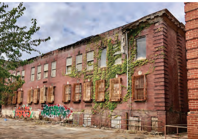
Rubell Museum DC before renovations
