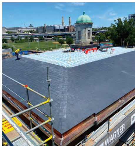
New slate roof system under construction
