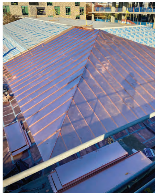
New standing-seam copper roof system in progress
