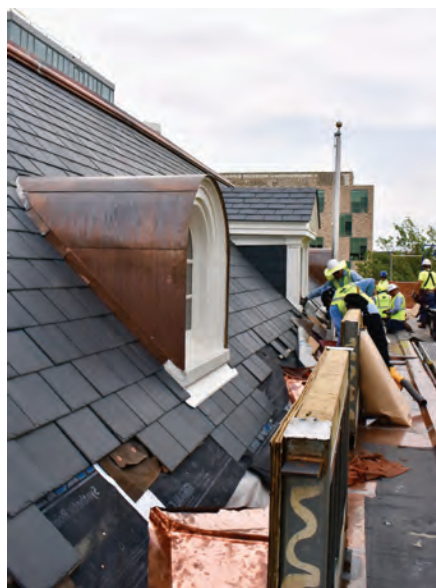
Wagner Roofing craftsmen fully restored 12 dormers.
