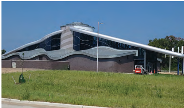
Korellis craftsmen custom-bent fascia metal pieces to accommodate radius, concave and convex perimeters.
