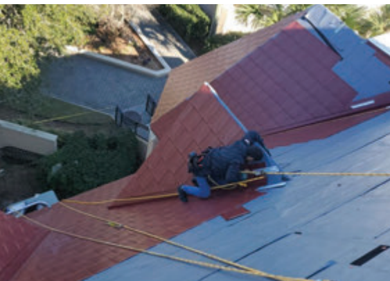
A Reliant Roofing team member installs new metal shingles.
