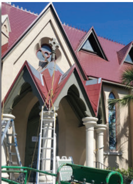
The church's main sanctuary's roof presented a host of architectural complexities with its myriad steep-slope sections and dormers.
