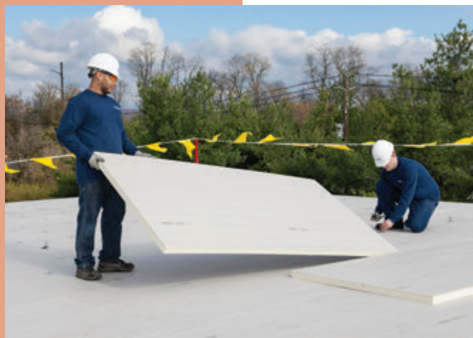
Polyisocyanurate roof insulation is available in varying thicknesses to meet project-specific performance requirements
