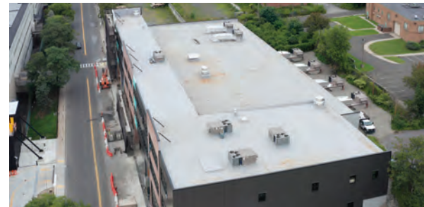
The studio’s new roof system
