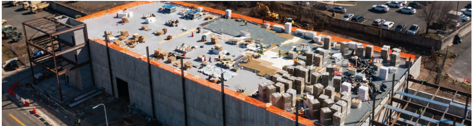
Initial work on the studio's roof
