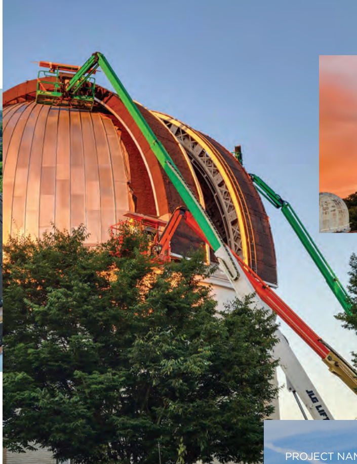
Left to right: Workers used the dome's apex as a tie-off point; 7,000 square feet of tapered and curved standing-seam panels and 1,100 square feet of flat-lock panels were installed on the dome; a close-up of the dome's new panels
