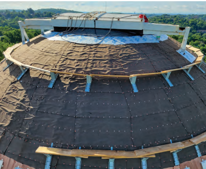
Left to right: Workers used the dome's apex as a tie-off point; 7,000 square feet of tapered and curved standing-seam panels and 1,100 square feet of flat-lock panels were installed on the dome; a close-up of the dome's new panels
