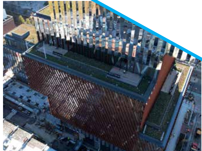
Aerial view of one of the vegetative roof systems
