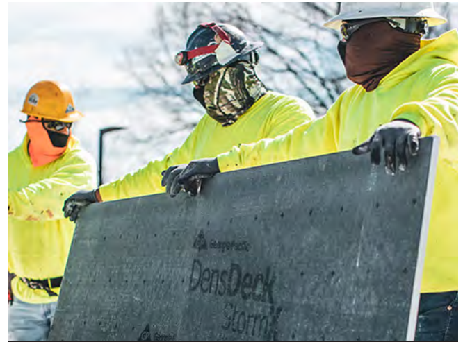
DensDeck® StormX™ Prime Roof Board was the first gypsum cover board to be FM classified for Very Severe Hail (VSH) in approved single-ply membrane assemblies.
