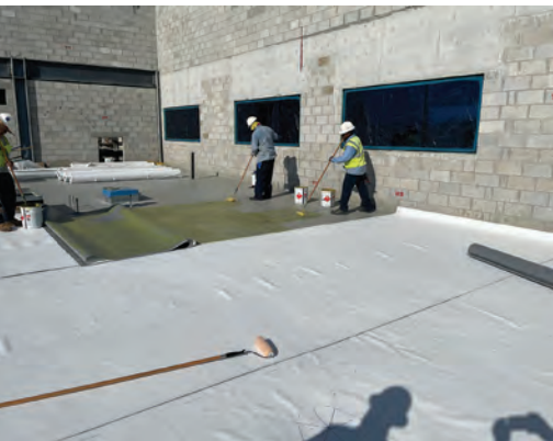
Workers adhere TPO membrane as a temporary roof.
