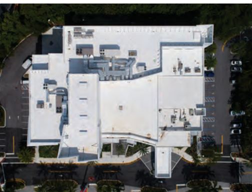
Aerial view of the theater's new roof system
