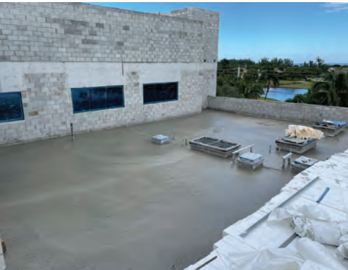
Lightweight insulating concrete was used in some areas.
