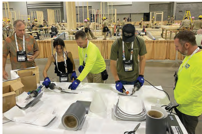
Volunteers from Johns Manville, Denver, demonstrate the initial steps of welding a T-patch.
