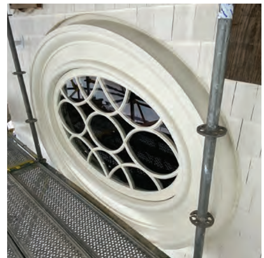
A newly renovated window
