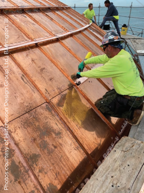
Left to right: New roof drains to direct rainwater to an interior copper gutter system were installed around the dome's base; a worker locks a standing-seam panel to a lower panel.
