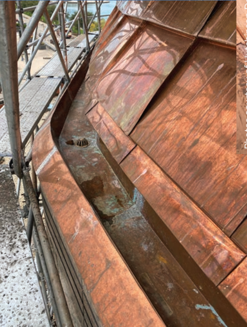
Left to right: New roof drains to direct rainwater to an interior copper gutter system were installed around the dome's base; a worker locks a standing-seam panel to a lower panel.
