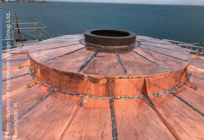
Left to right: Entrance to Adler Planetarium; flared transitions in copper panels on top of dome; aerial view of the planetarium's new copper roof
