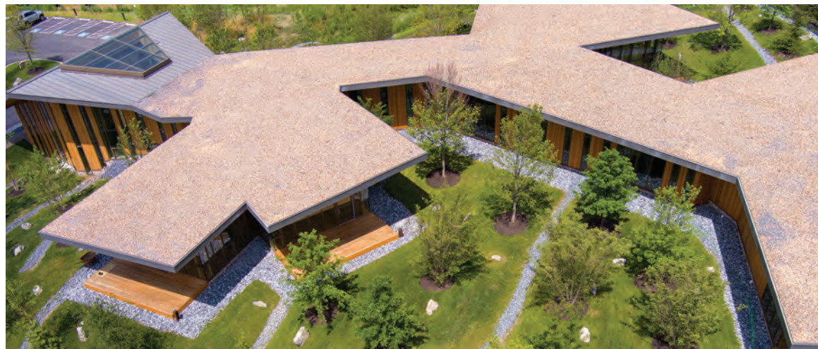
Clockwise from top left: The building owner wanted a rusted patina look for the metal roof, so Houck Services used PAINT GRIP; Timberlite lava rocks were incorporated in other roof areas for aesthetic purposes; about 5,000 holes were drilled into edge metal to achieve an artistic look of icicles during winter.
