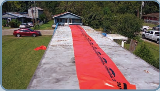
The roof in the process of being Stormsealed
