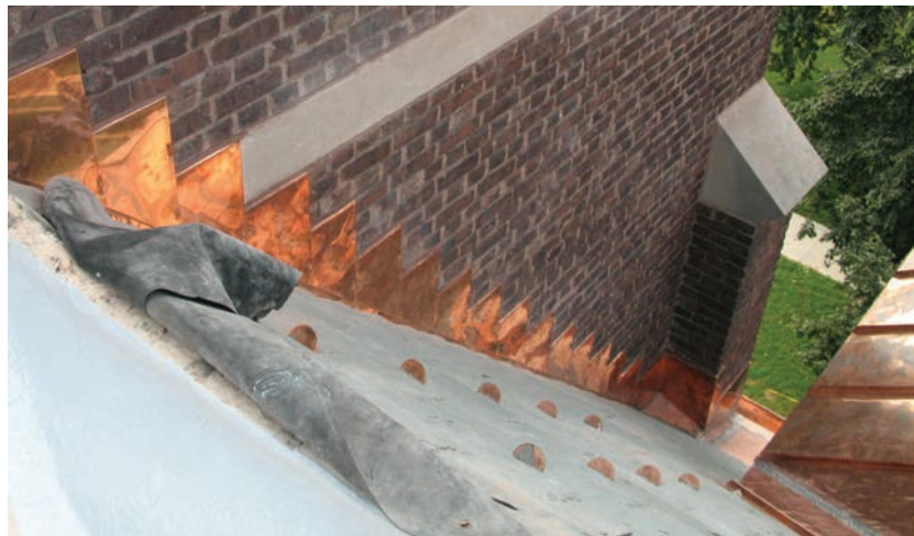
Photo 5: Regularly sized steps in counterflashings help improve their appearance, especially where masonry units are of uniform size.
