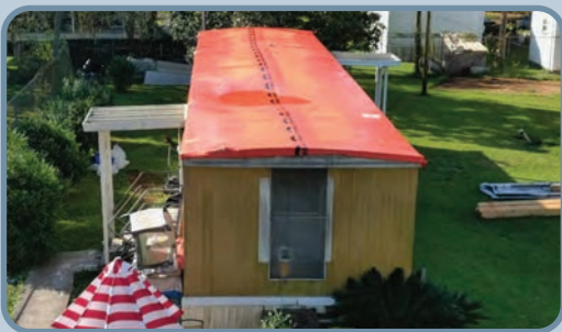
The roof after Stormseal installation
