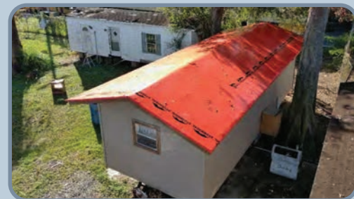
After Stormseal installation
