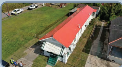
After Stormseal installation
