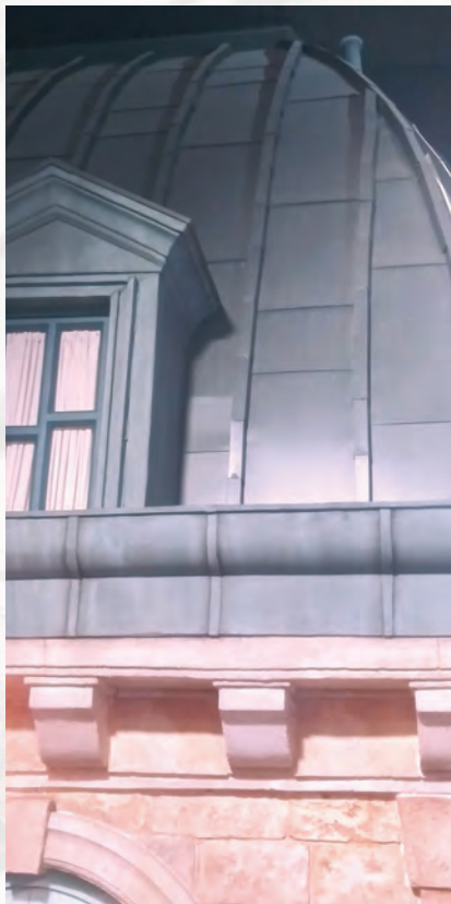
All the zinc panels for the attraction's interior roof, gutters, drains, chimney and crown molding were custom-made by P.A. Roofing and Sheet Metal craftsmen.
