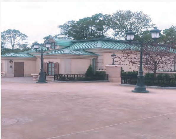
On the roof over the restrooms, P.A. Roofing and Sheet Metal craftsmen roll formed convex and concave standing-seam titanium zinc panels.
