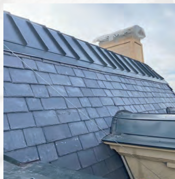
Composite slate was used for the exterior roof.
