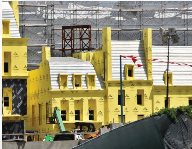
Exterior metal roof decks under construction
