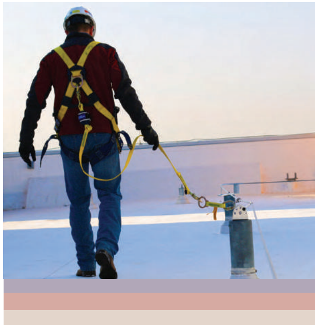
Horizontal lifeline systems are an example of travel restraints.
