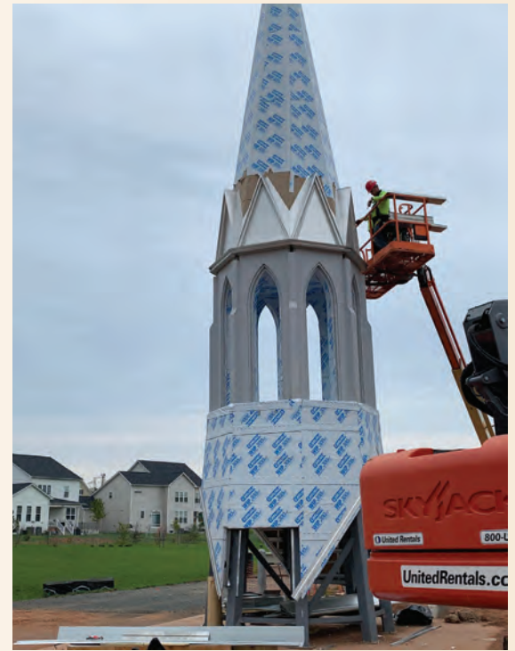
A major part of the roofing project included a 57-foot-tall steeple.
