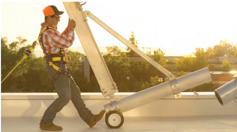
An example of a fall-arrest system: a worker wearing a harness with a self-retracting lifeline connected to certified anchorage.
