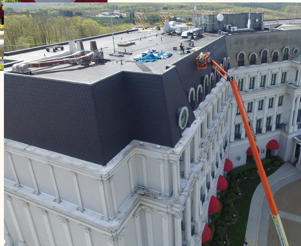
Workers install new synthetic slate
