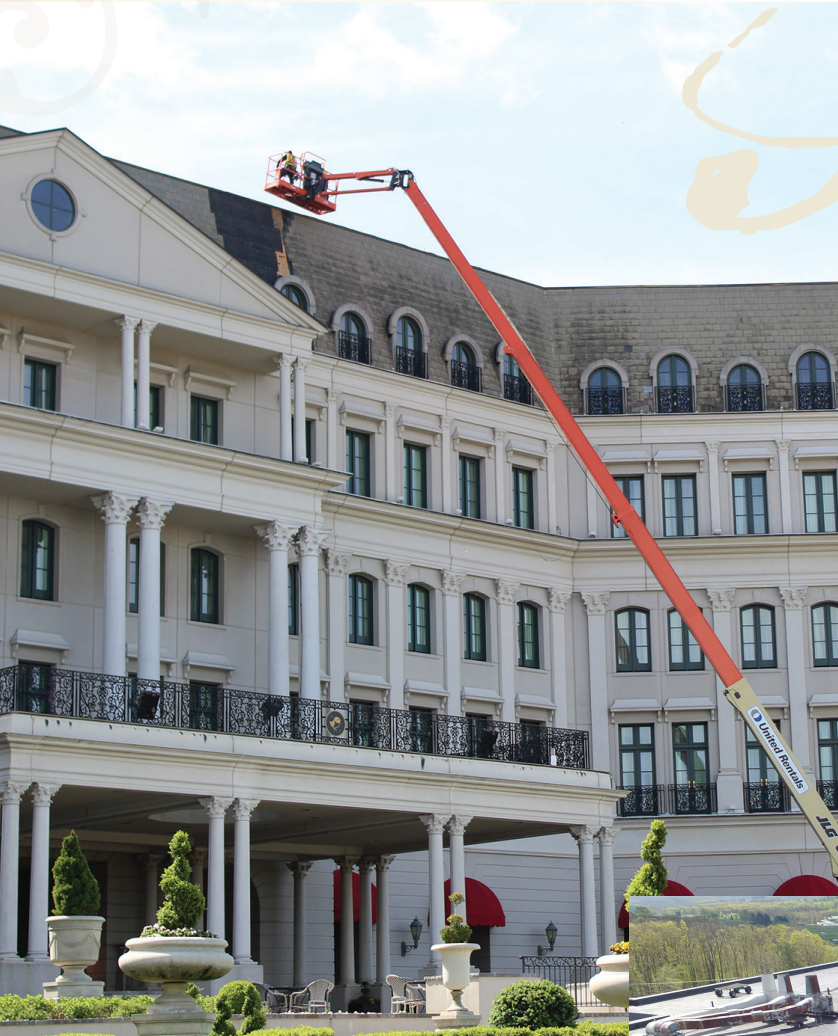
Workers divided into three crews to tackle the reroofing project.
