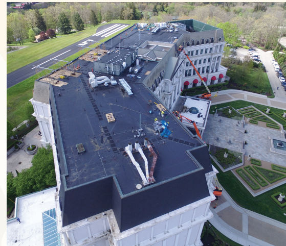
An aerial view of the roof under construction
