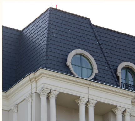
The new mansard roof
