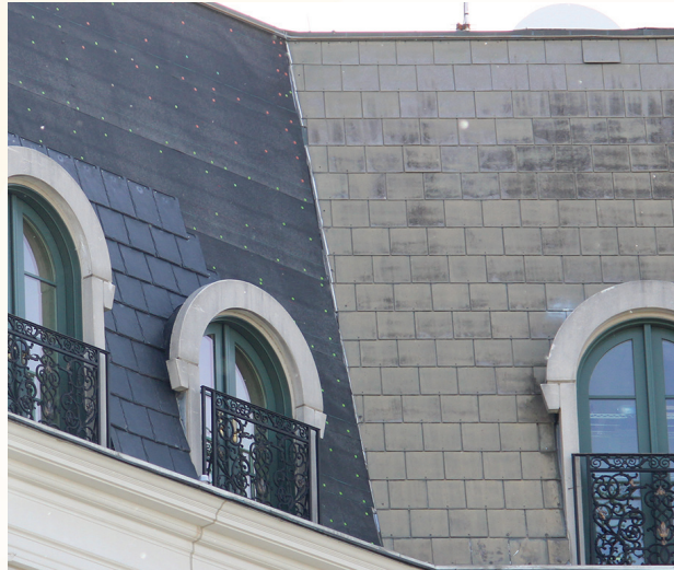
The mansard roof during construction
