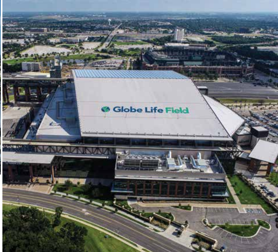
From opposite page left to right: More than 19,000 tons of steel were used to build the roof; the 5.5-acre retractable roof weighs 24 million pounds; about 2,000 people worked more than 6 million man-hours to build the venue in 30 months.
