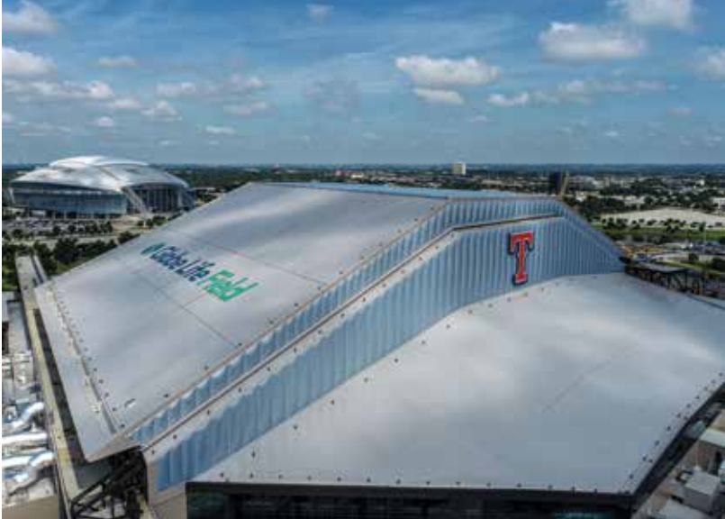
From opposite page left to right: More than 19,000 tons of steel were used to build the roof; the 5.5-acre retractable roof weighs 24 million pounds; about 2,000 people worked more than 6 million man-hours to build the venue in 30 months.
