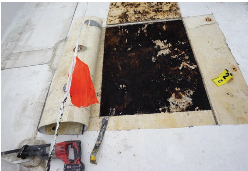
Photo 3: Another investigative opening made into a soft roof in a northern climate shows a gypsum cover board present. Both the gypsum cover board and oriented strand board roof deck are saturated and cannot support any load. Effectively, only the single-ply roof membrane is preventing people from falling through.
