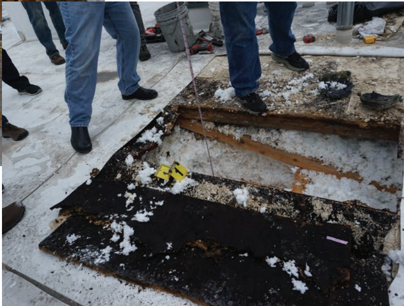
Photo 2: An opening made during an investigation into the cause of soft roof areas. The openings were made in winter. The oriented strand board (black in the foreground) is saturated. This is the same roof system as Photo 1.
