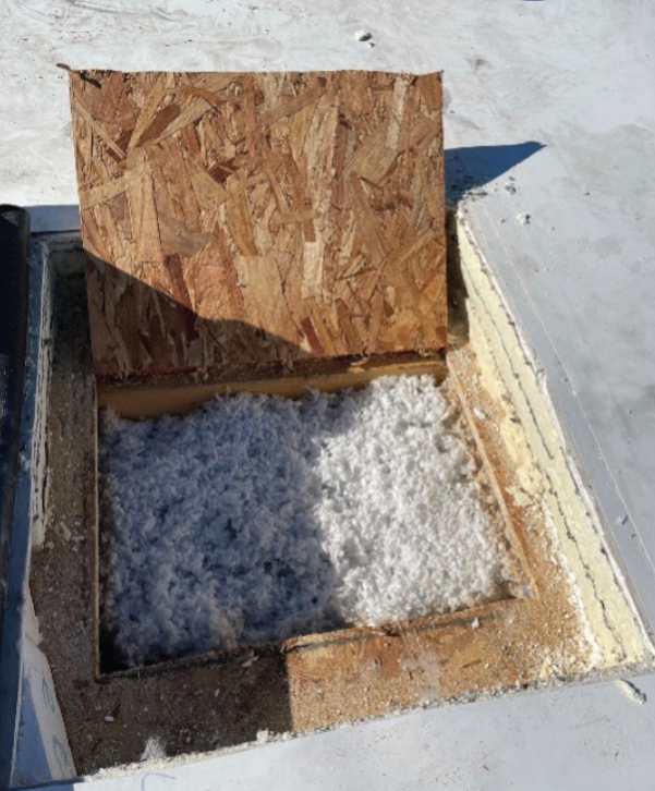
Photo 4: A view of a cold roof in a northern climate with blown insulation. There are numerous soft spots and decayed decking throughout this roof. However, in areas like this where a polyisocyanurate saddle is installed between drains, the oriented strand board is in pristine condition.
