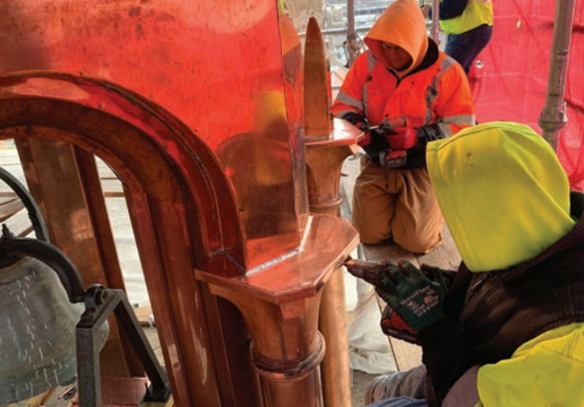
F.J.A. Christiansen Roofing craftsmen re clad a dome in copper.
