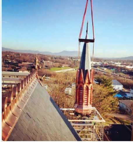
The spire was restored using 20-ounce copper.
