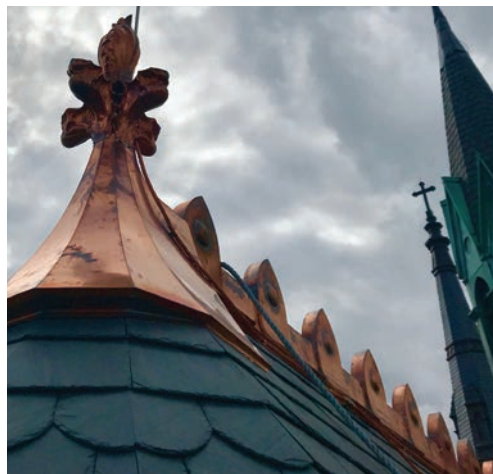
Left and right: The crew replicated and replaced each piece of copper.
