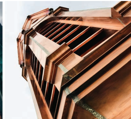
The roof could not withstand scaffolding weight, so the spire was lowered to the ground for restoration.
