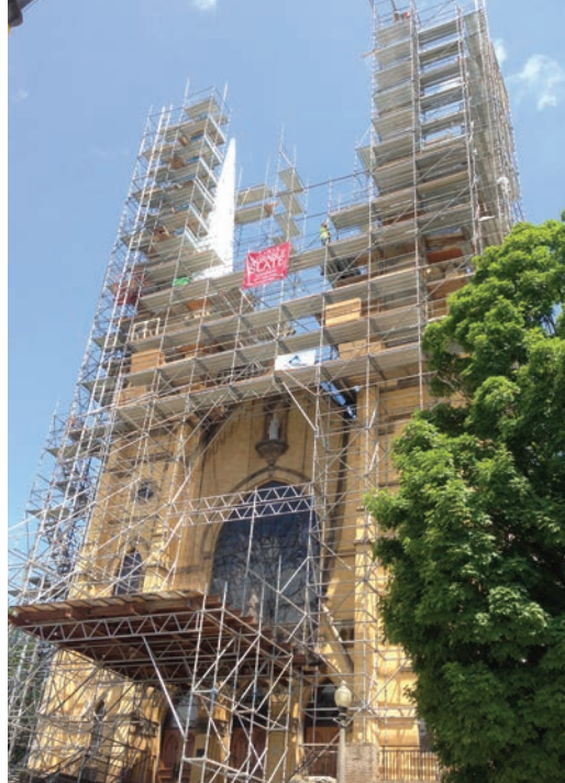
Scaffolding was erected around the steeple.
