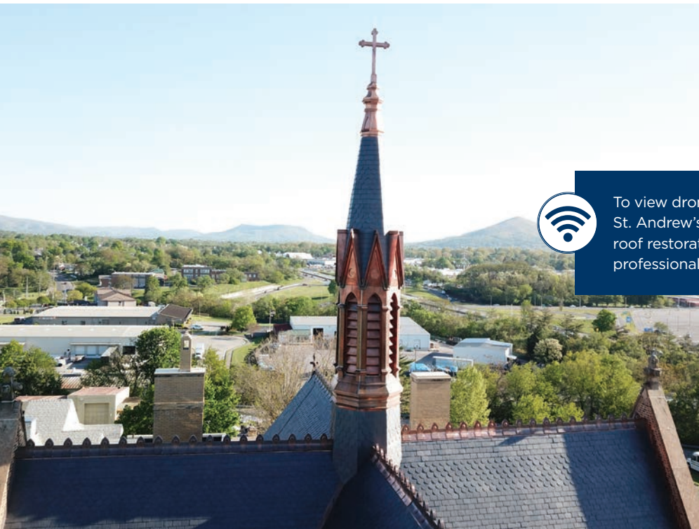
The newly restored roof system and spire
