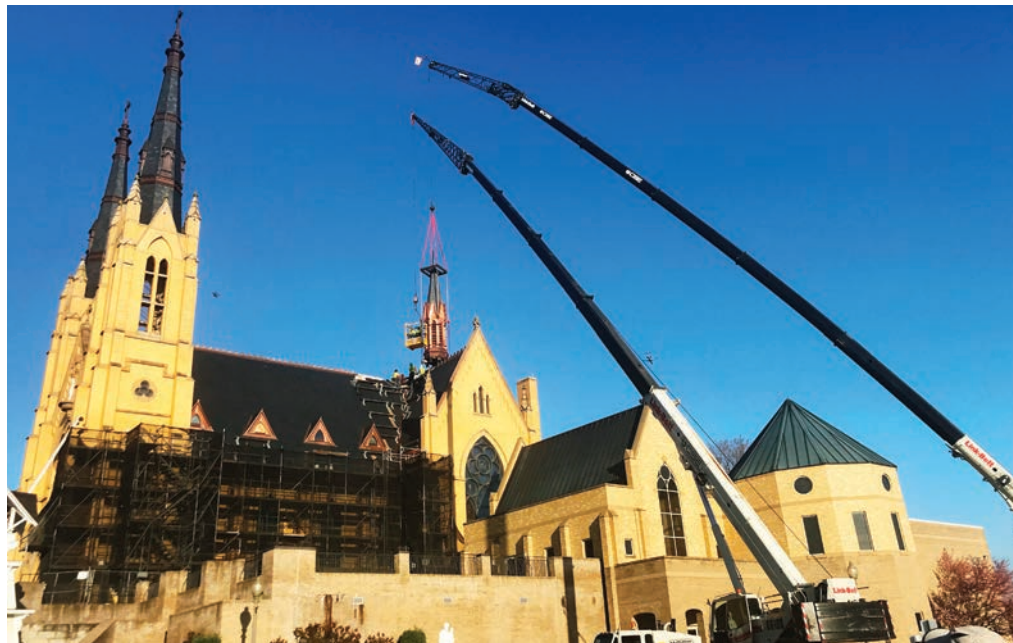
The roof could not withstand scaffolding weight, so the spire was lowered to the ground for restoration.
