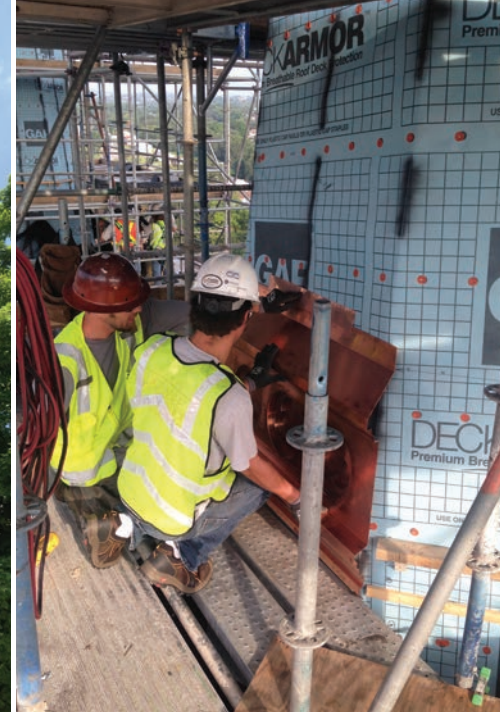
Workers clad the spire in customized copper.
